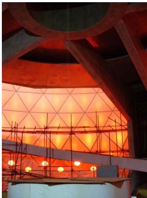
The inner skin and spiral ramp inside the Matrimandir (photo: Julian Lines).
